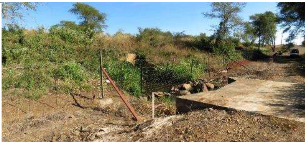
One culvert connecting upper stream area with lower stream area
