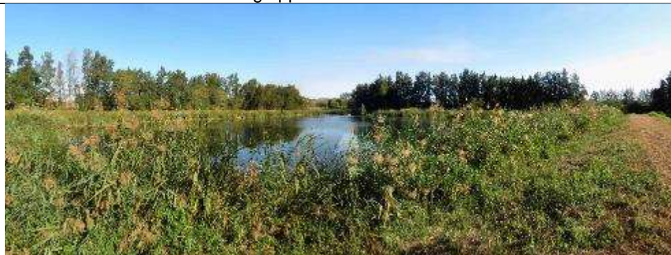
Dam in drainage line
