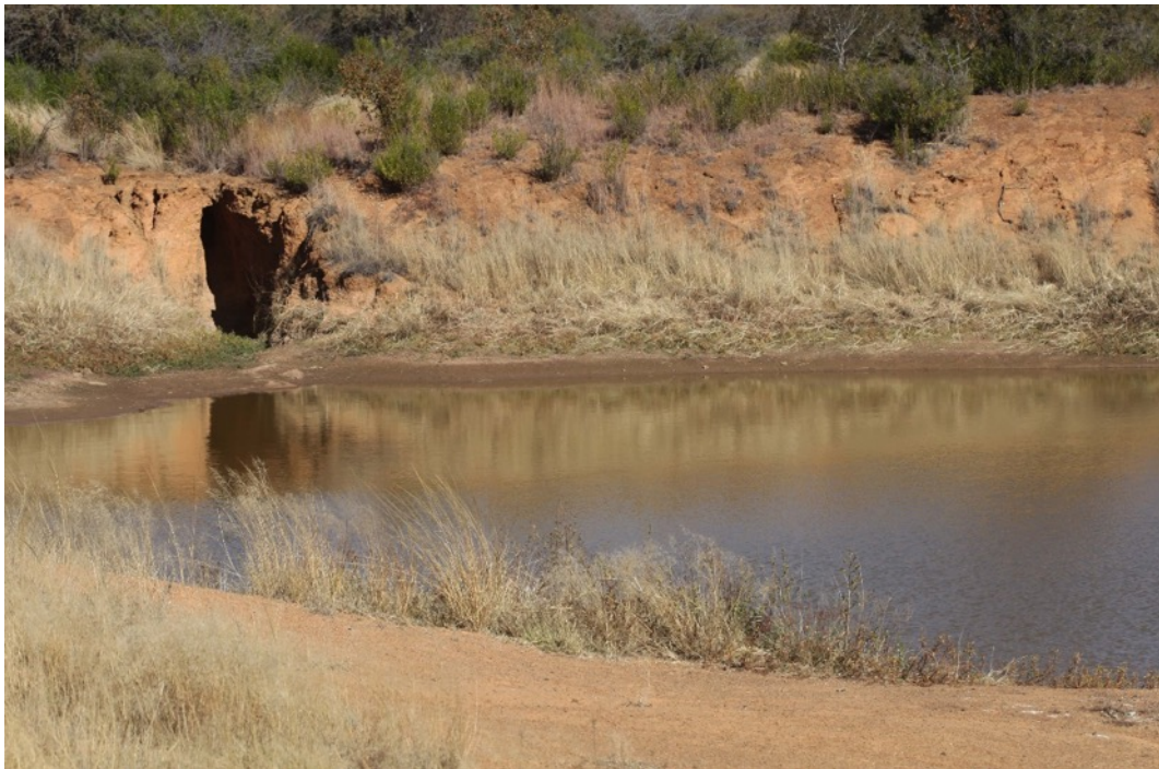
Photo 14 Dam 6 at the site. Groundwalls with sparse vegetation are prone to be eroded. Photo: R.F. Terblanche
