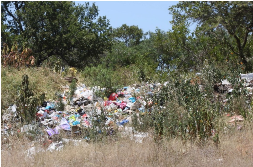
Photo 16 Some parts of the groundwalls at Dam 6 at the stie, are covered by rubble owing to informal dumping.
