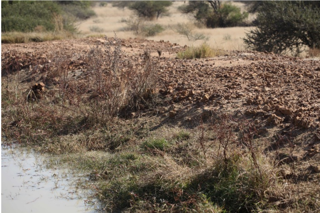
Photo 13 Groundwall at Dam 4 at the site. Photo: R.F. Terblanche.
