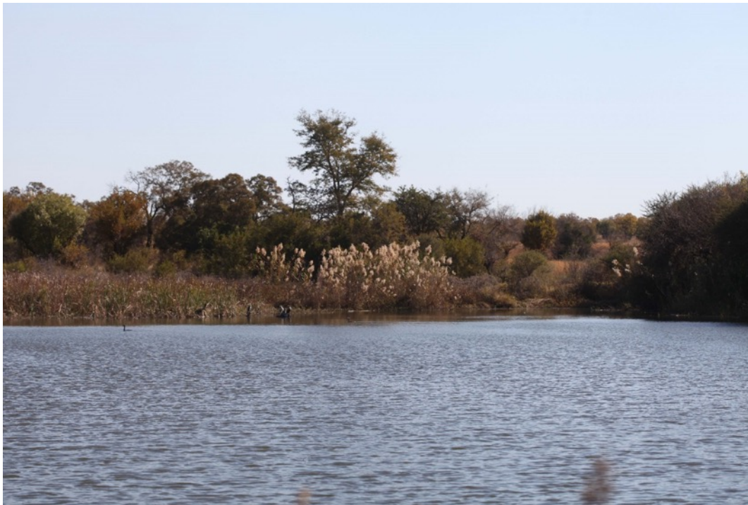
Photo 9 The largest dam, Dam 1, near the northern boundary of the site. Photo: R.F. Terblanche.
