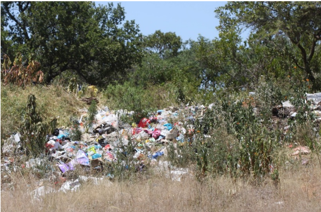
Photo 9 Some parts of the groundwalls at Dam 6 at the stie, are covered by rubble owing to informal dumping. Photo: R.F. Terblanche
