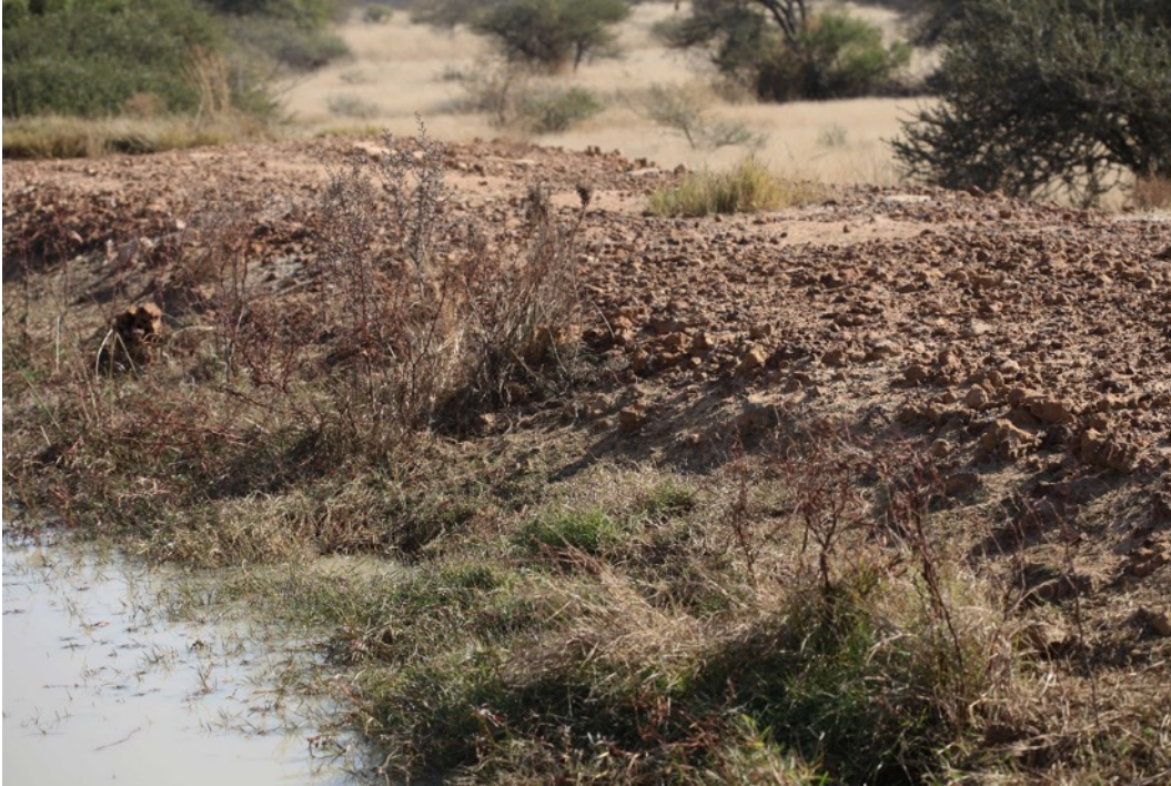
Photo 6 Groundwall at Dam 4 at the site. Photo: R.F. Terblanche.
