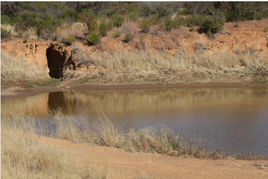
Photo 7 Dam 6 at the site. Groundwalls with sparse vegetation are prone to be eroded. Photo: R.F. Terblanche
