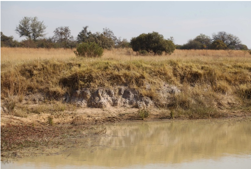
Photo 5 Part of Dam 4 at the site. Photo: R.F. Terblanche
