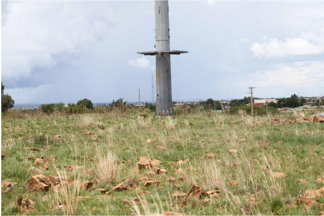
Photo 17 View of rocky ridge and tower at Erf 6149 Jouberton. Photo: R.F. Terblanche.
