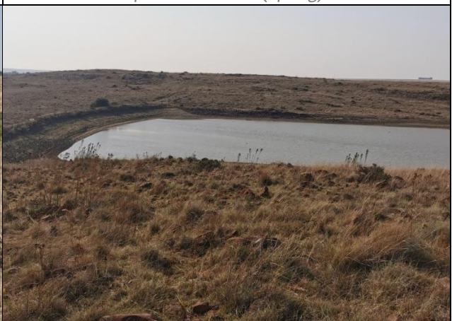
Figure 25: Man-made dam along watercourse.
