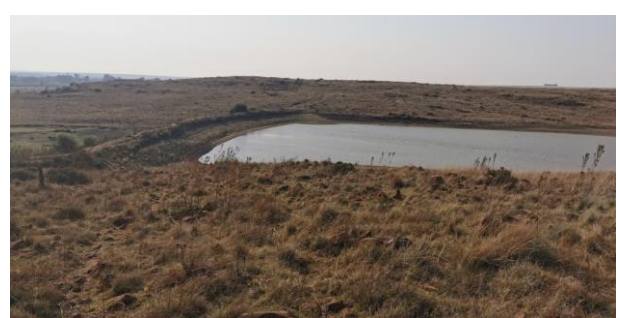
Figure 25: Man-made dam along watercourse.
