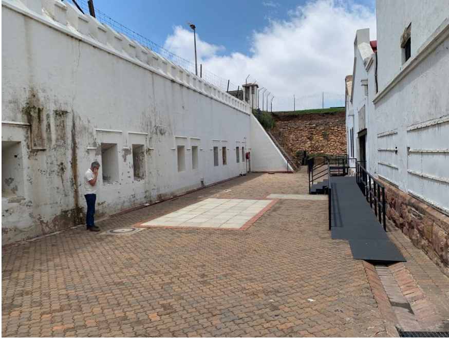
1. West Elevation looking North
