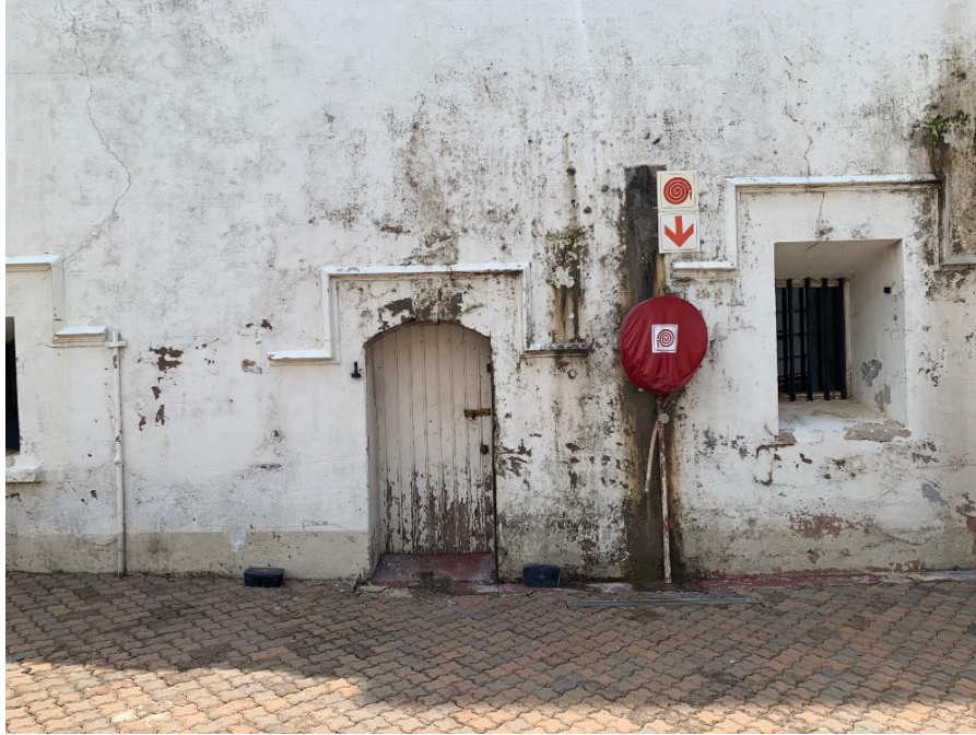
3. Entrance door on West Elevation
