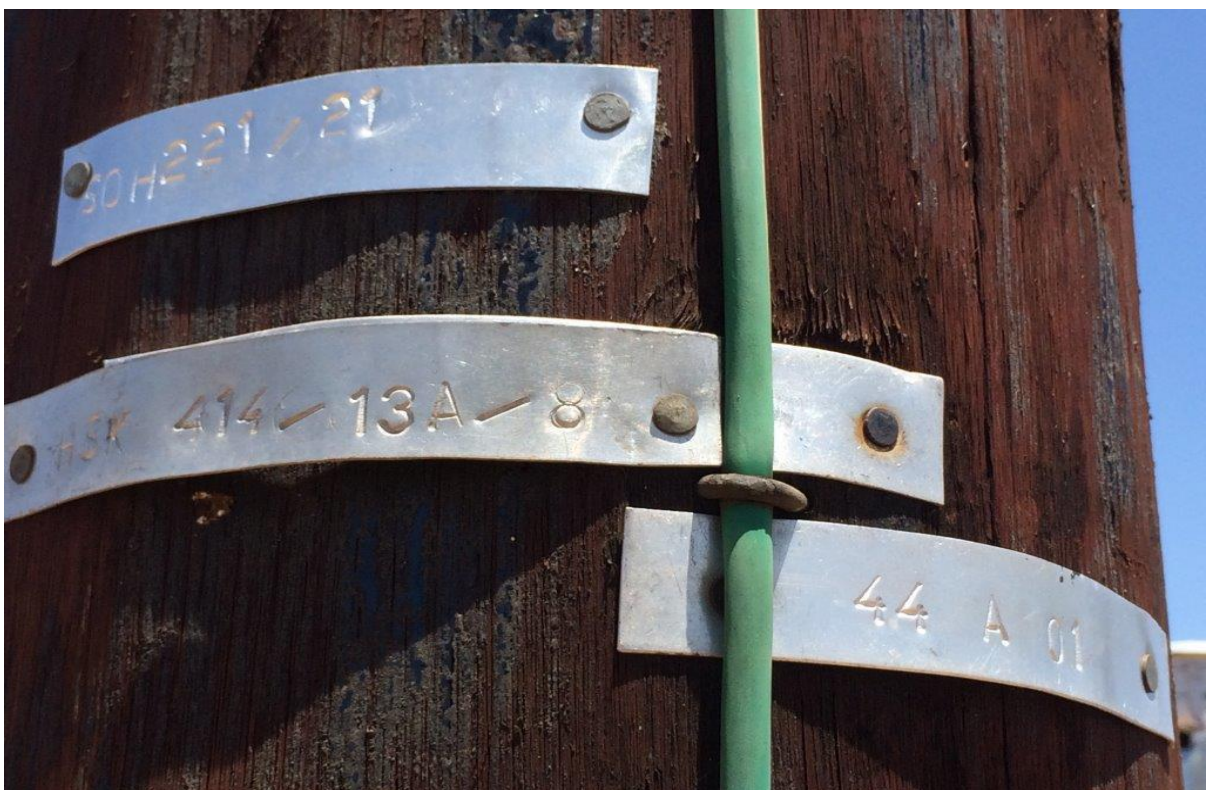
Picture 6: Shows the existing pole numbers on site
