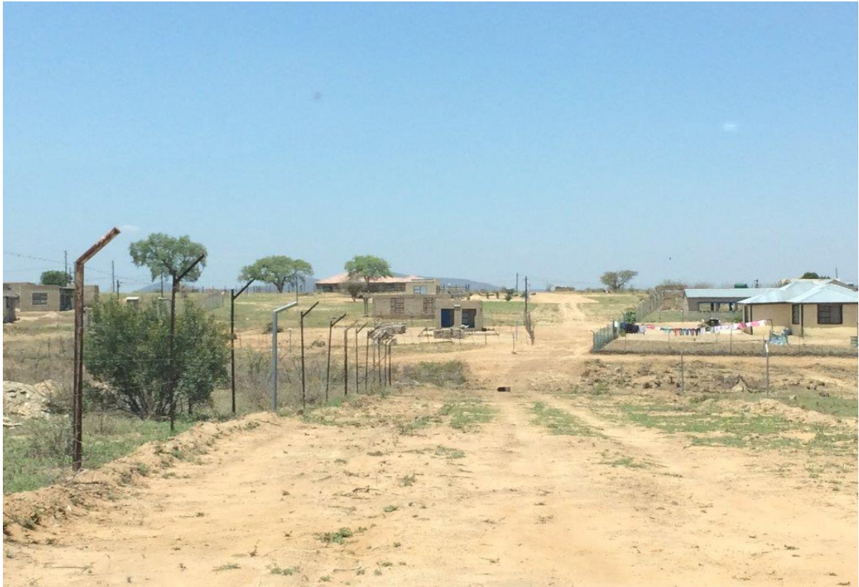
Picture 3: Shows the houses to be electrified in the village
