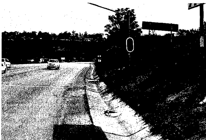
Fig 6: Existing road edge SW channel and catchpits along eastern edge of Pitts Avenue-R55 (Gautrans K71.02)
