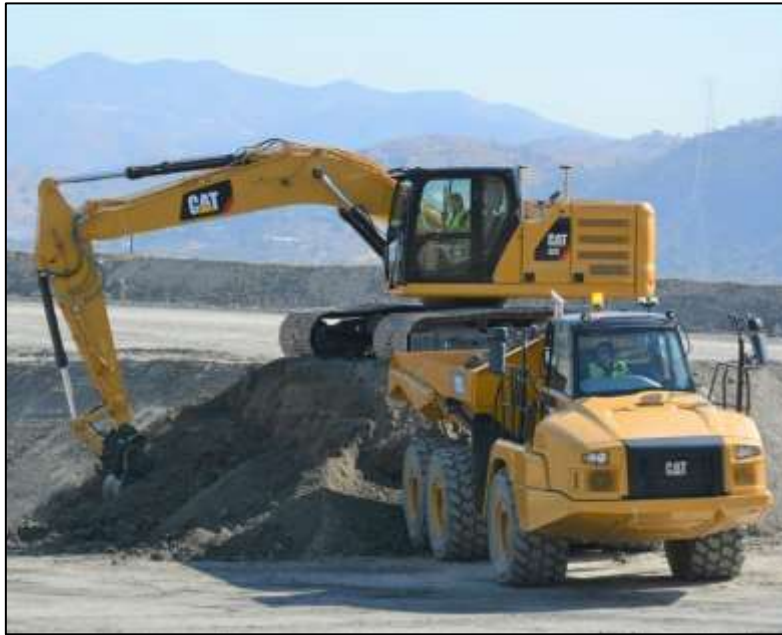
Figure 8. Overburden Removal with Truck and Shovel
