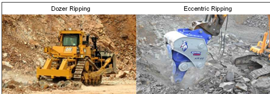
Figure 9. Overburden Removal with Ripping
