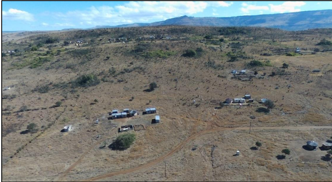
PHOTOGRAPH 1: THOKOZA ACCESS ROAD UPGRADE PROJECT
