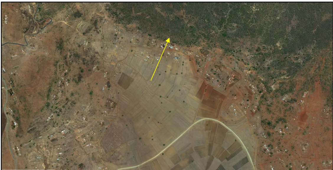
PHOTOGRAPH 3: NOTE THE CHANGE IN THE VEGETATION COMPOSITION FROM DEGRADED GRASSLAND TO BUSHVELD
