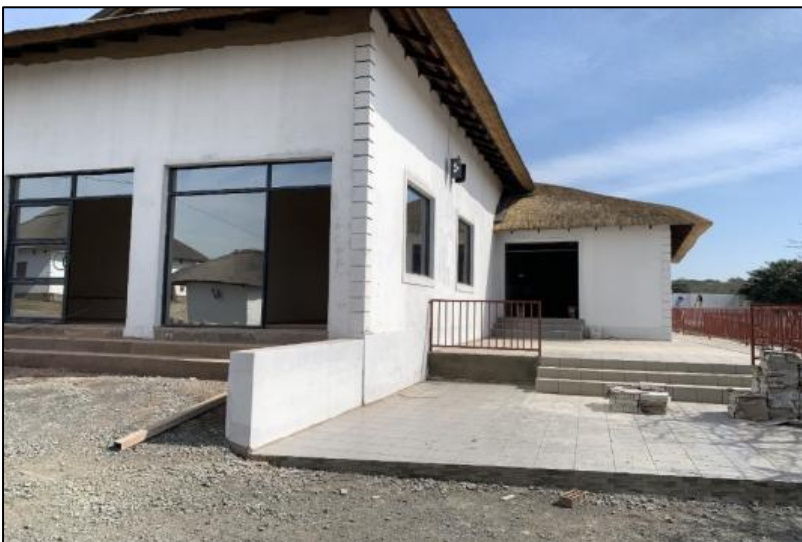
Plate 2: View of the buildings being constructed.
