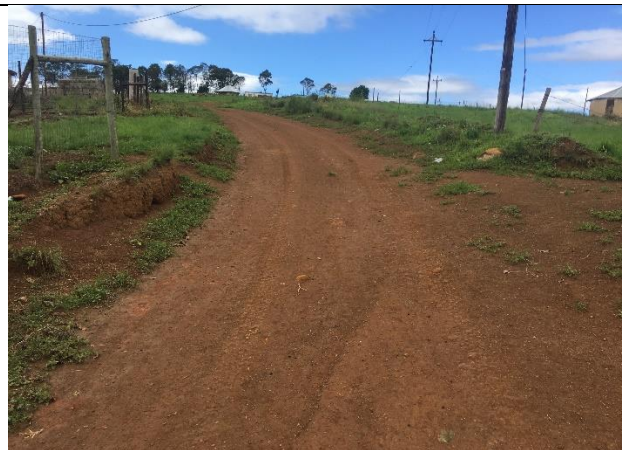
Plate 4. Image looking south west along existing track amongst existing residential dwellings, proposed for road upgrade.
