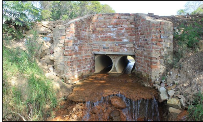
Figure 5-2: The newly constructed culvert crossing (TBC, 2022)
