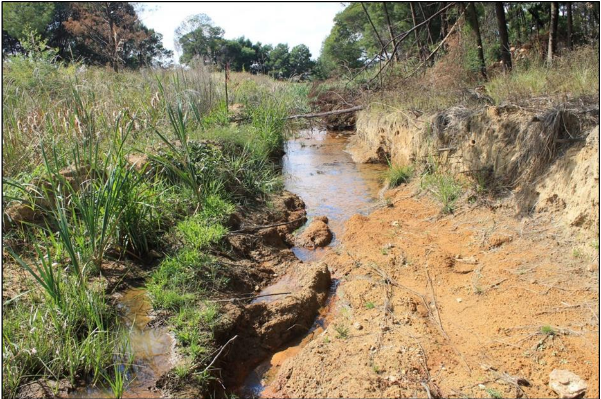
Figure 4-18: Erosion at Site PT1 (TBC, 2022)
