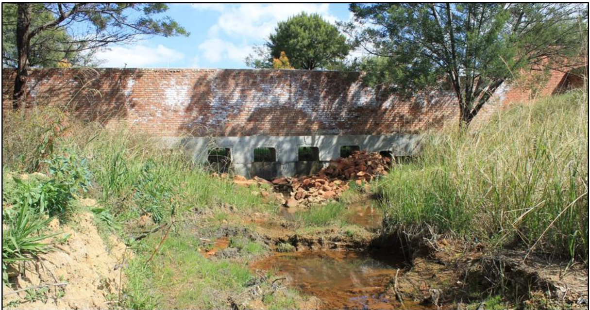
Figure 4-17: Instream Wall and Rock dump on site
