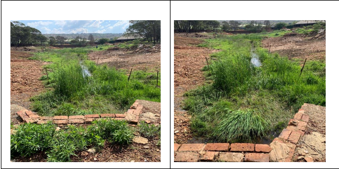
Figure 2-5: Building rubble removed from the floodline
