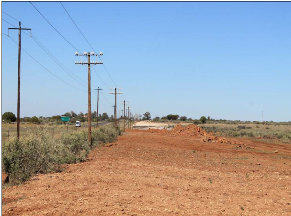
Plate 1: The site (taken towards the south)
