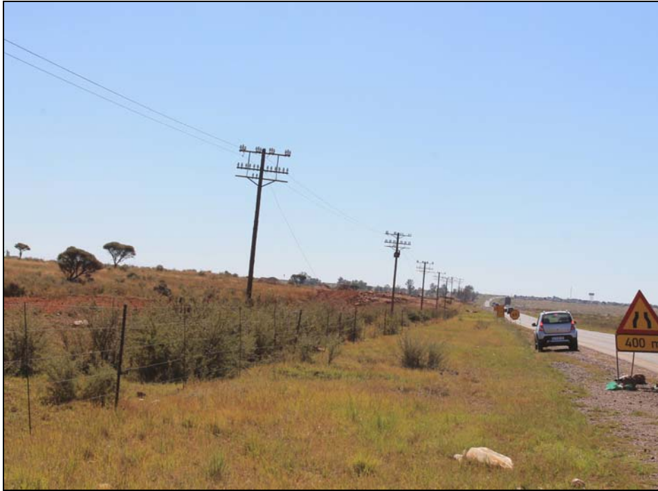
Plate 13: The existing access road (N18) towards Vryburg (taken towards the north)
