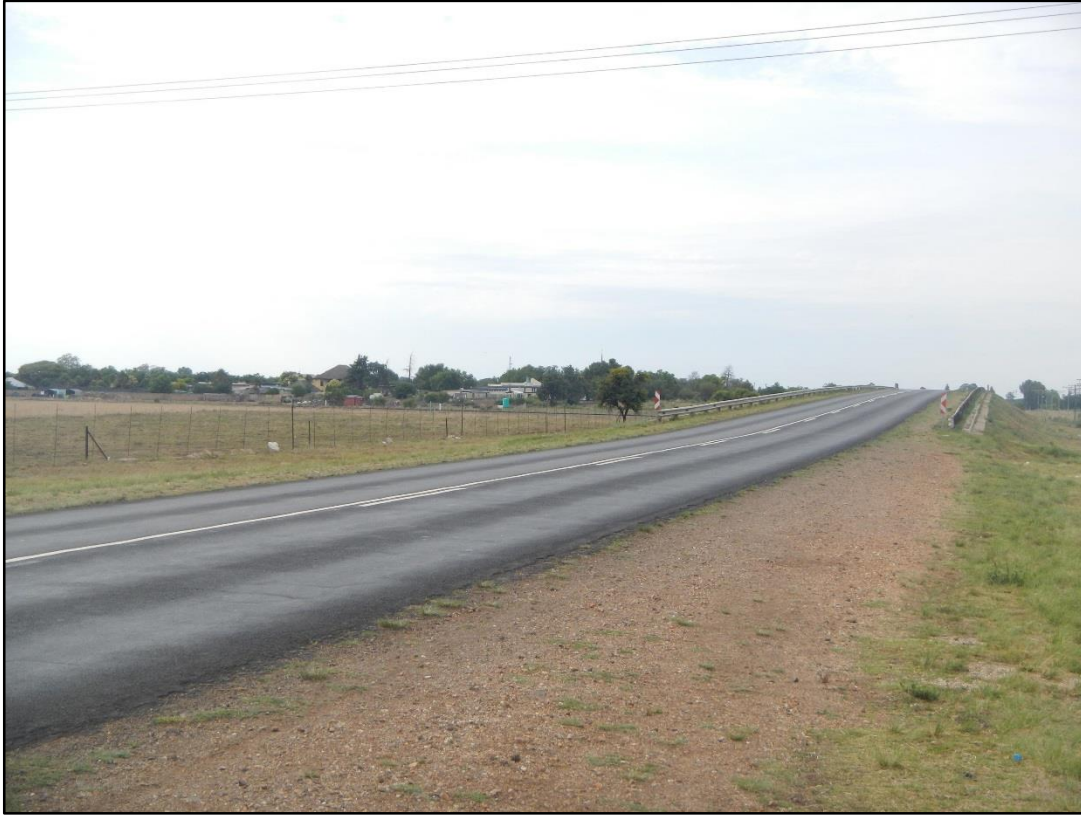
Figure 12: Outskirts of the town of Lichtenburg which comprises a mix of commercial, light/service industrial and residential development
