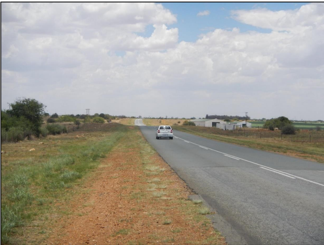
Figure 5: R505 main road which traverses the corridor in a north-west to south-east direction
