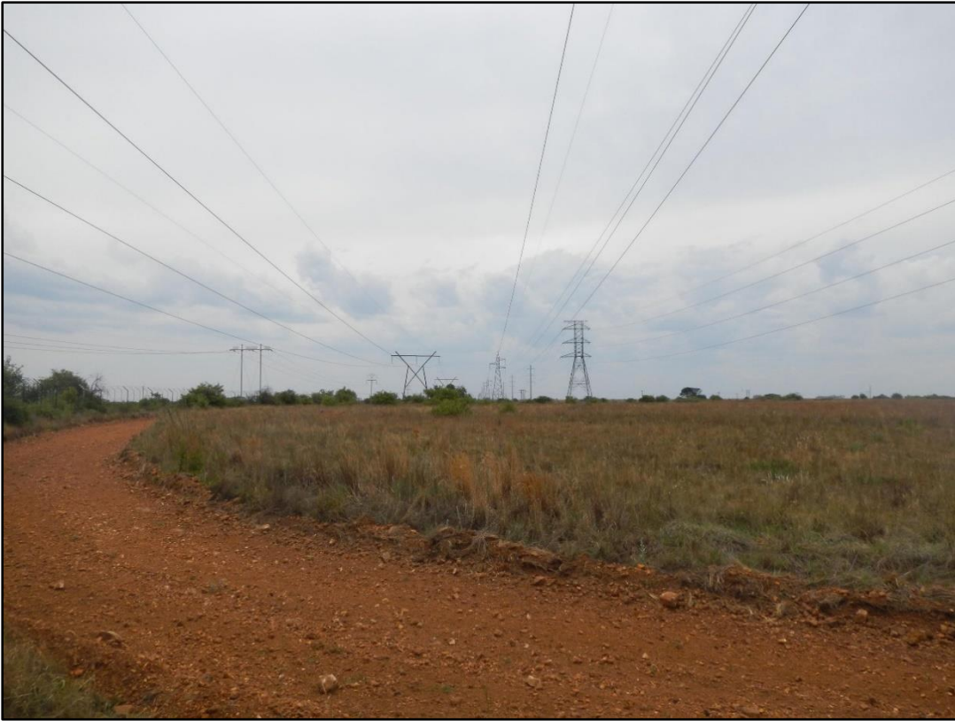
Figure 10: View from the proposed power line corridor showing the relatively natural character of the area, as well as the existing 132kV power line which the proposed power line corridor will follow
