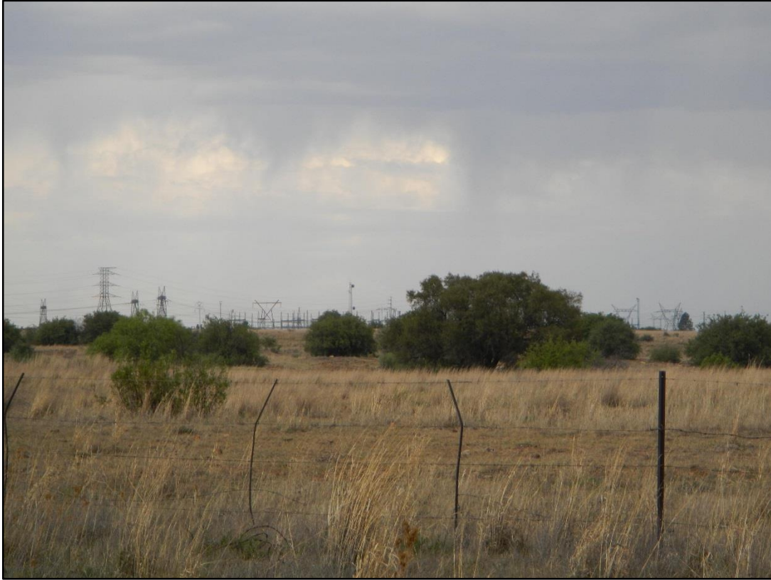
Figure 11: Tall steel structures that make up the Watershed MTS, as well as the tall steel towers of the existing 132kV power lines that run to the Watershed MTS, which can be seen from various parts of the study area
