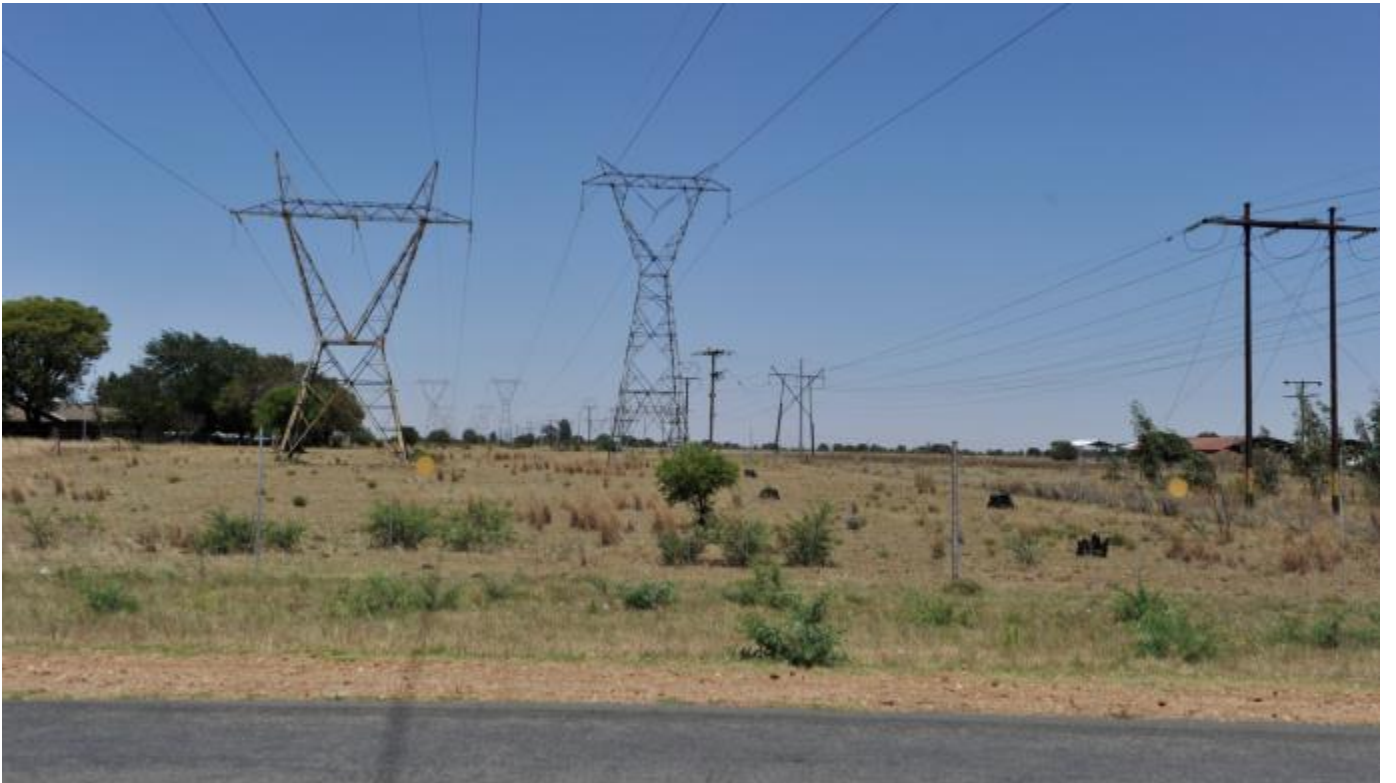
Figure 4: Existing high voltage lines in the study area.
