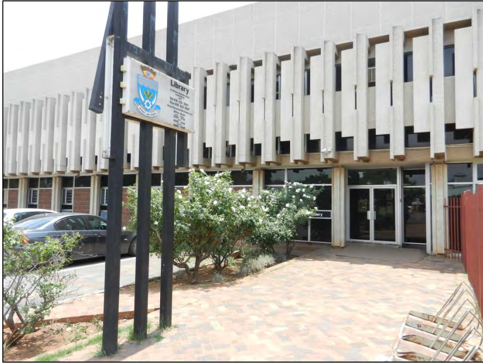
Figure 1: Ditsobotla Public Library, Nelson Mandela Drive, Lichtenburg
