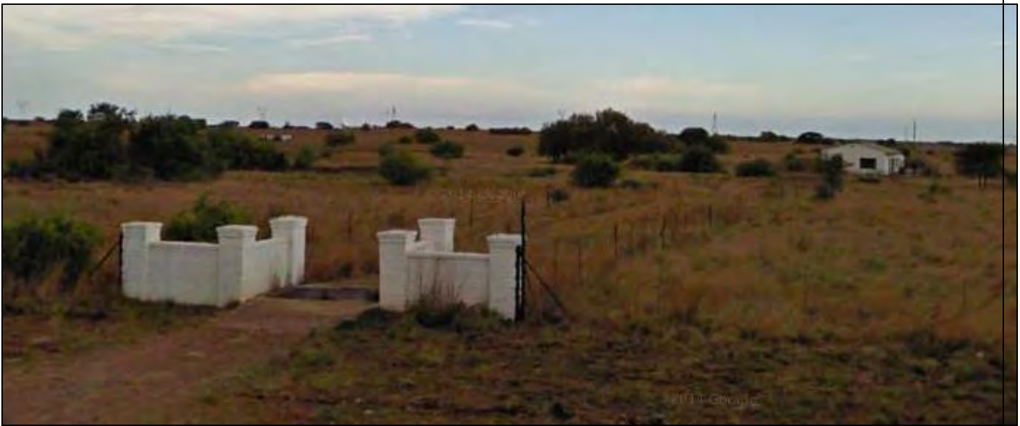
Figure 6: Eastern entrance to Houthaalbomen (PV Site) - off the R505
