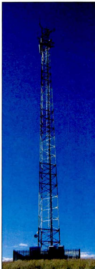
TYPICAL 3 LEGGED LATTICE MAST (PAINTED RED AND WHITE)
