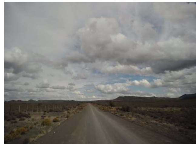
Photo 4: Southbound view along Biesiespoort Road (DR2405)
