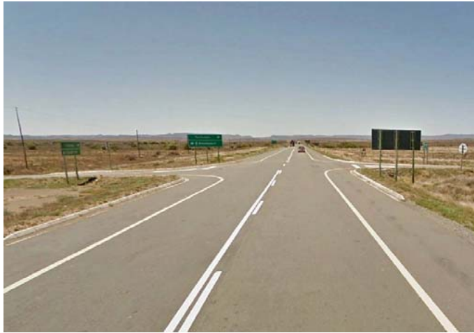
Photo 1: Northbound view along the N1 towards the R63 intersection
