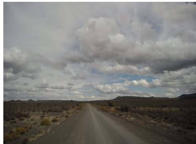
Photo 4: Southbound view along Biesiespoort Road (DR2405)
