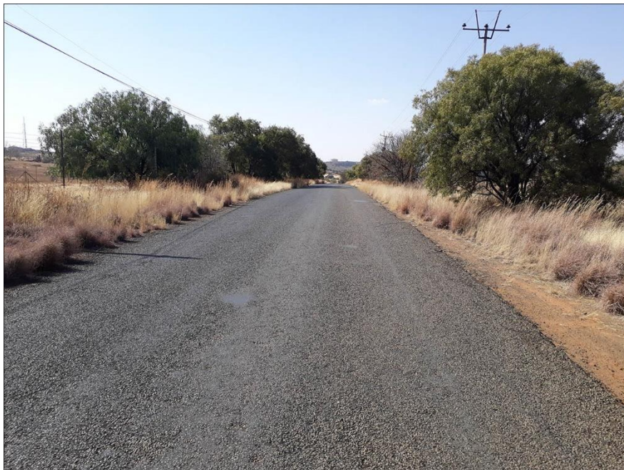
Sight distance to the North from Point 4
