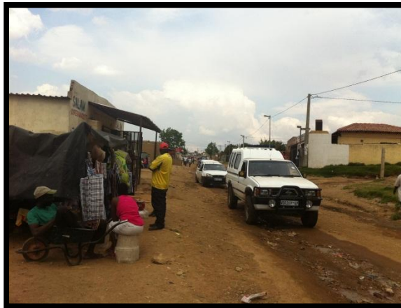
The road width of the gravel section that follows the paved road at William Nicol Drive is limited by farrows that have resulted from erosion and a series of rubbish dumps.
