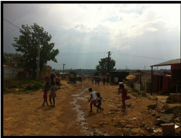
The road width of the gravel section that follows the paved road at William Nicol Drive is limited by farrows that have resulted from erosion and a series of rubbish dumps.
