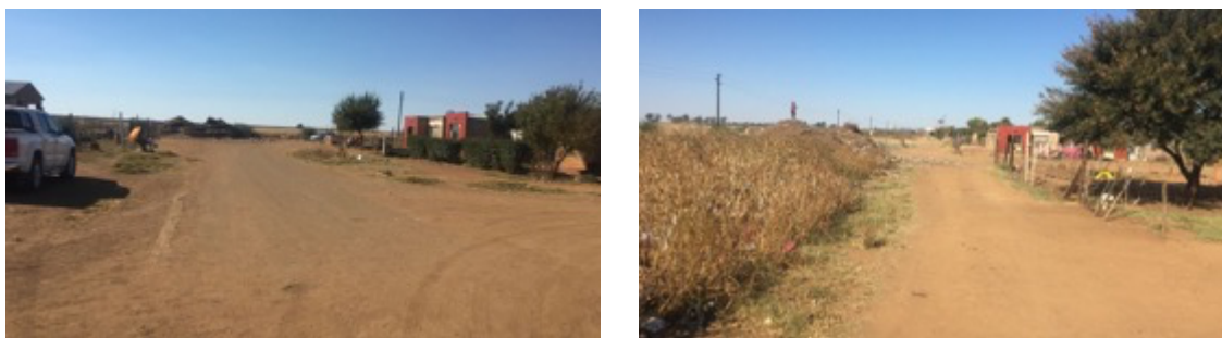
Figure 12– Intersection B – Road Condition
