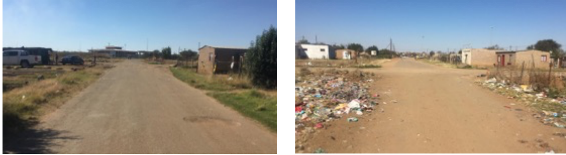
Figure 11– Intersection A – Road Condition
