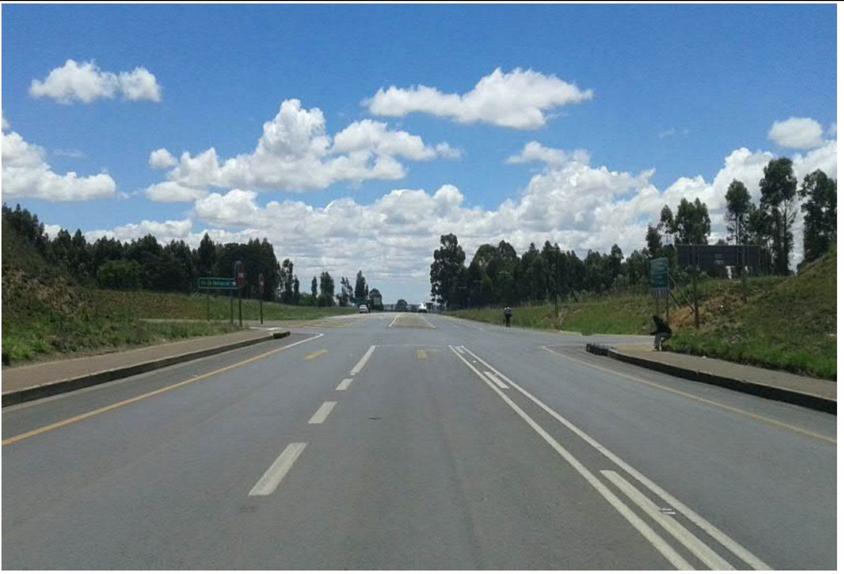
Road D1477 & N4 Offramp (facing north)
