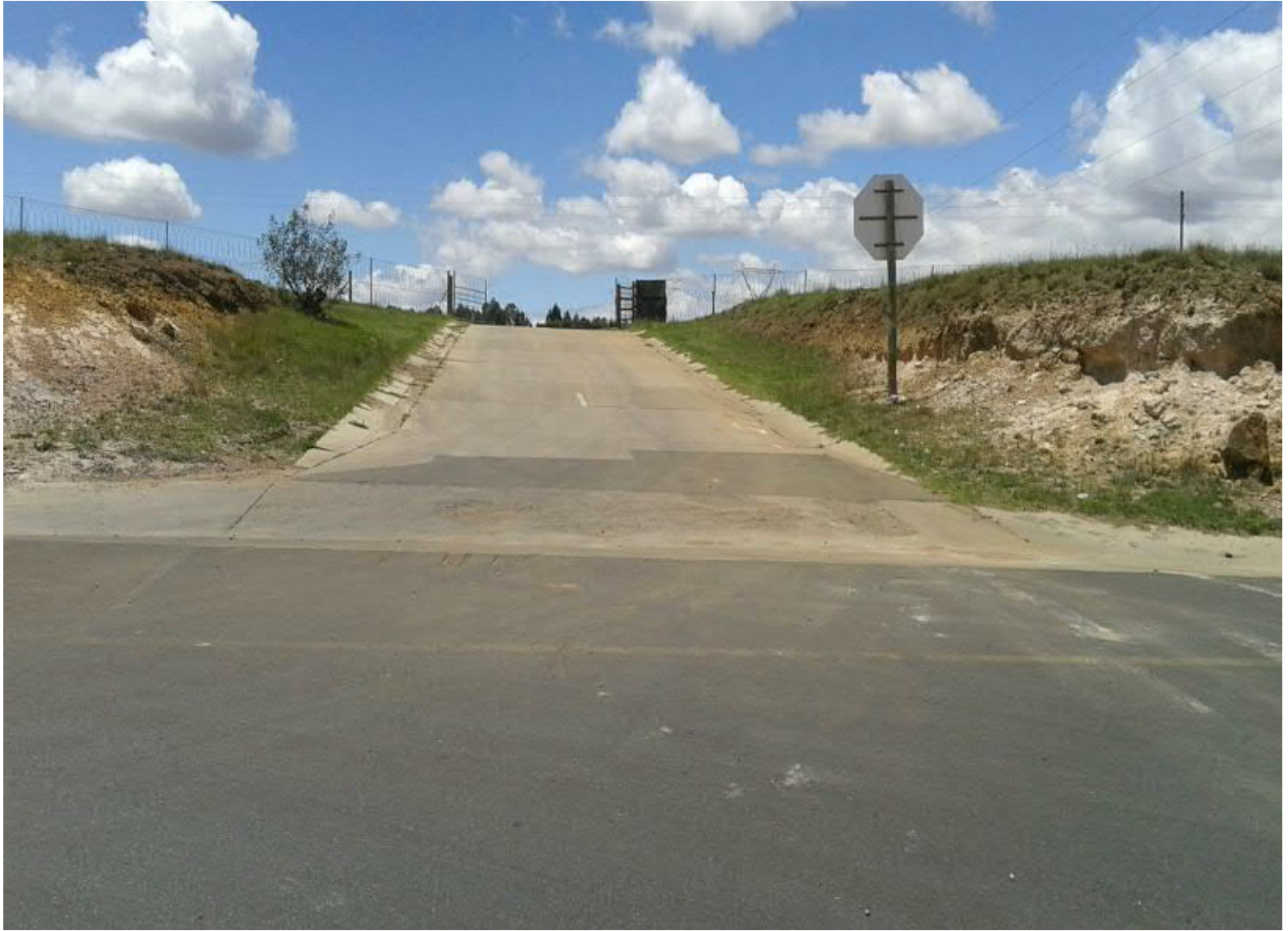
Road D1477 and Site Access 1 (facing east)
