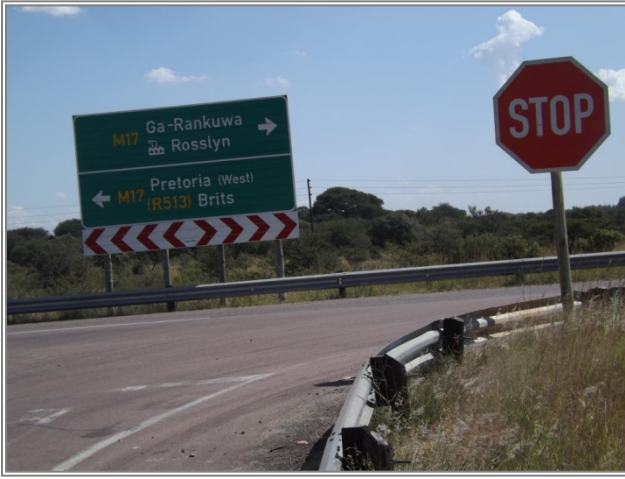
Southern ramp terminal M17 / N4 interchange
