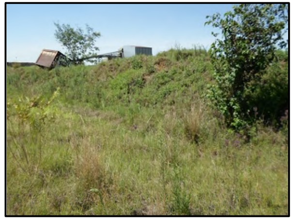
Figure 9. General site conditions
