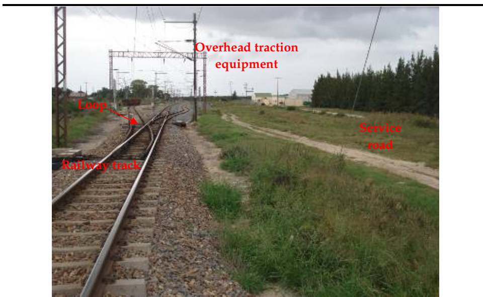
Figure 4.2 Typical Infrastructure Requirements for Rail Loop Upgrades
