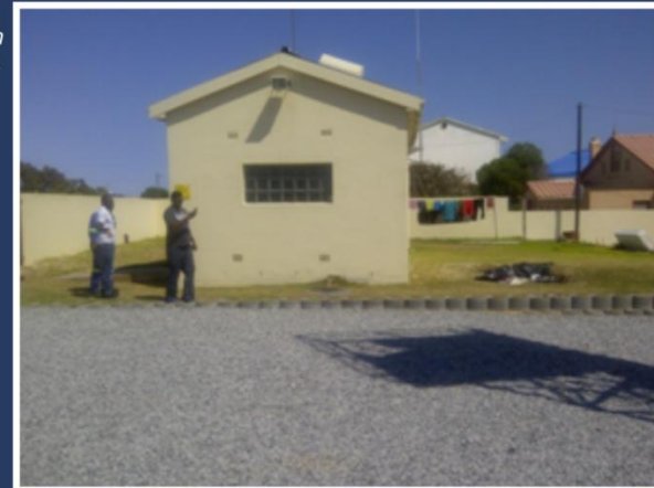
Figure 4: View of the existing engine room on ERF 45 which will connect to the new lighthouse.
