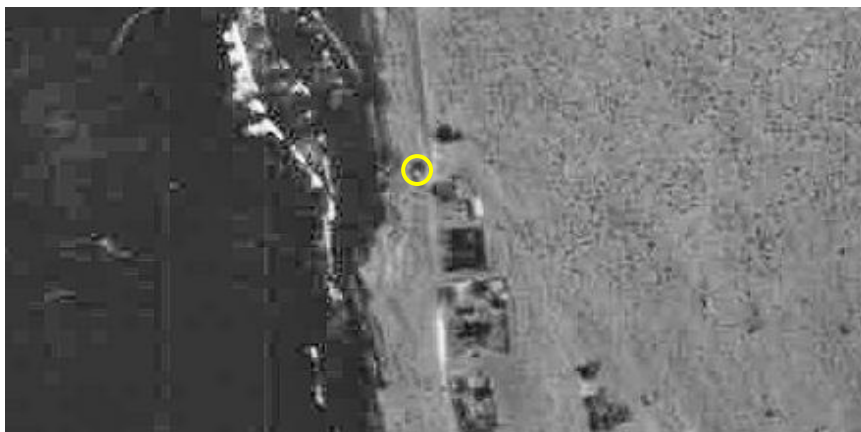
Figure 3 Excerpt from 1937 aerial photograph indicating the magazine. This is the only structure visible on the western side of Beach Street.
