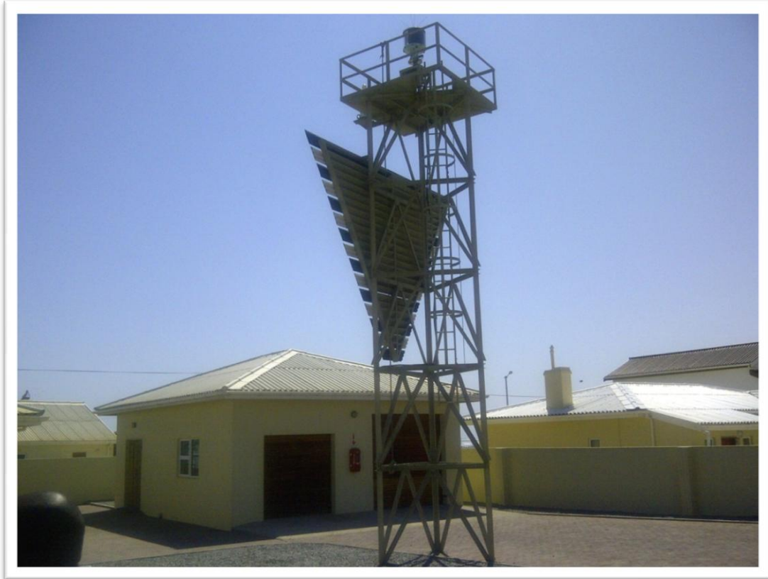
Figure 7-2 Existing lattice, aluminium lighthouse structure.
