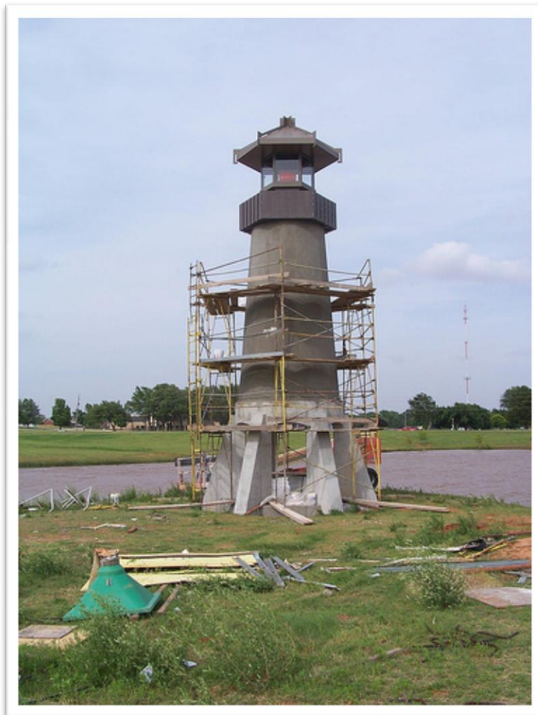
Figure 7-4 Example of a lighthouse ( Centennial Lighthouse ) under construction. (© K. Latham )
