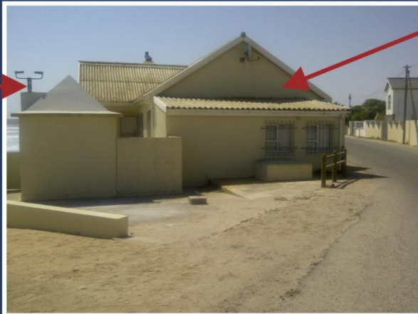
Figure 3: View of the site with the lean-to structure that will be demolished.
