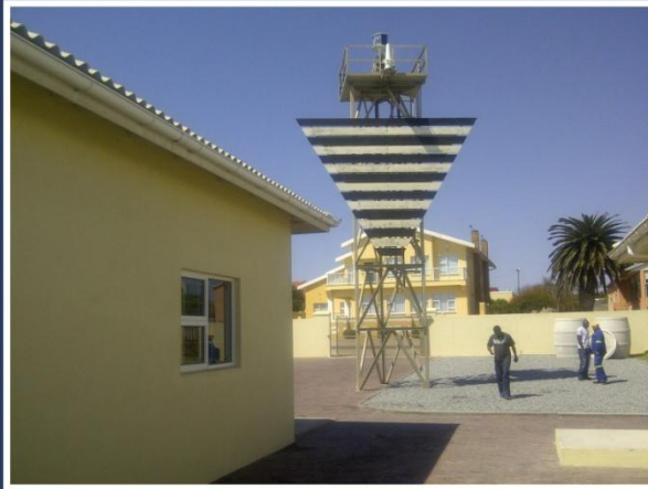
Figure 1: Front view of the existing lighthouse from Beach Street. This lighthouse will be decommissioned.
