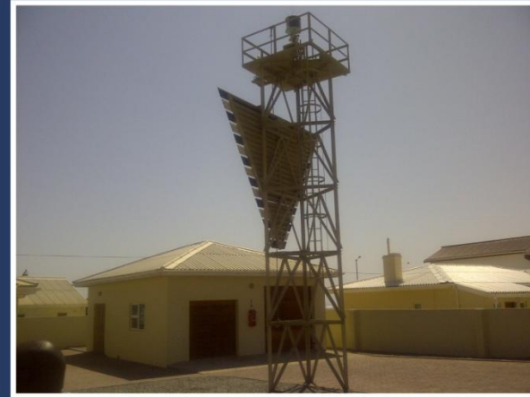
Figure 2: Side view of the existing lighthouse which will be decommissioned.
