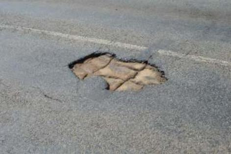
Figure 4.2: Pothole on the R545 road
