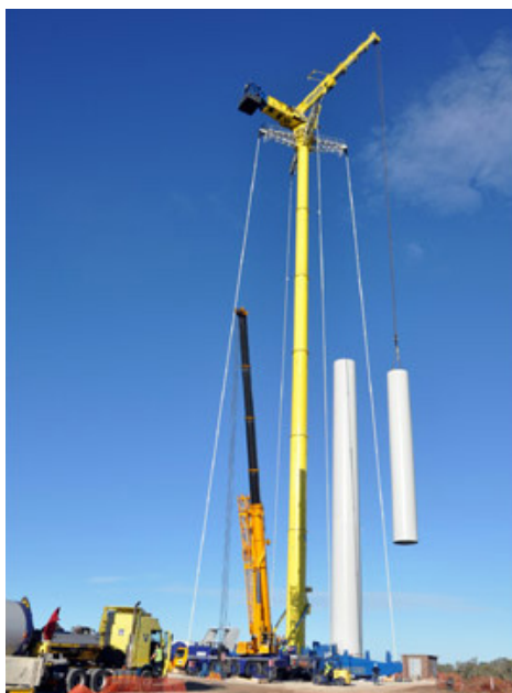
Figure 7: Cranes at work
