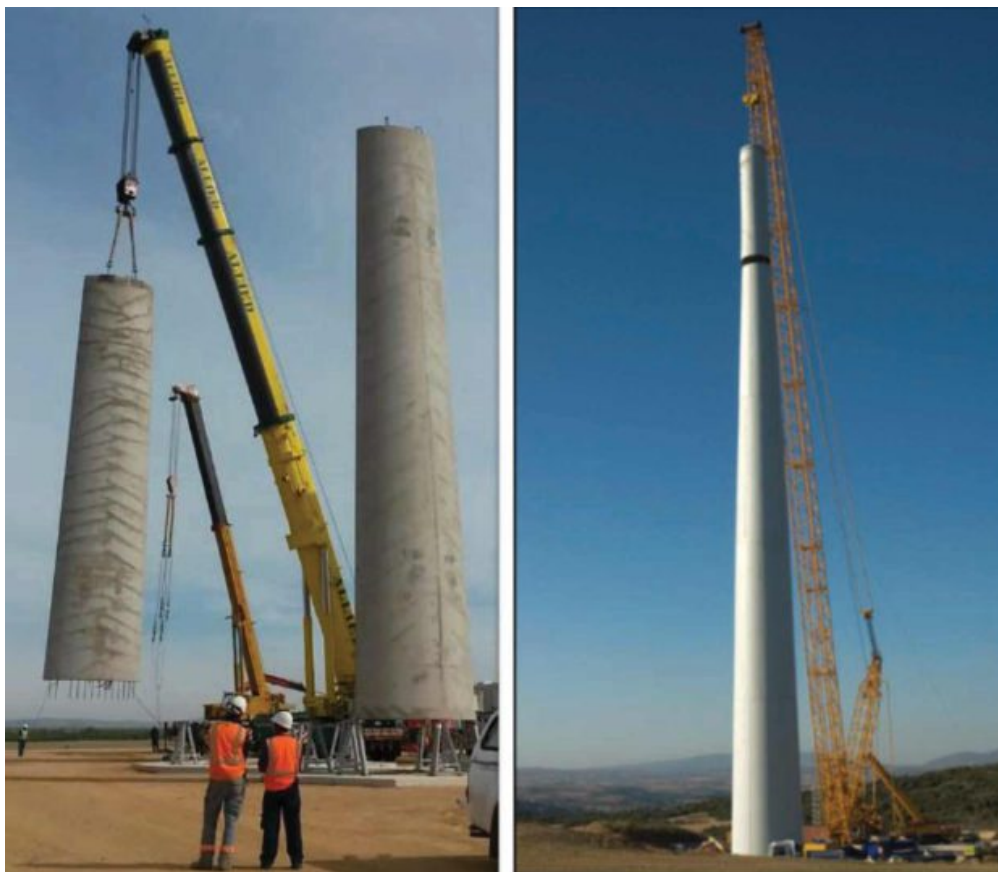
Figure 5: Concrete Tower Sections
