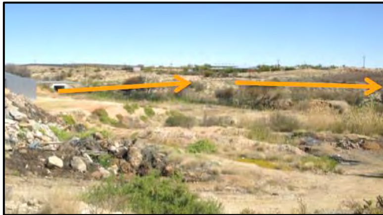
Figure 22: The section of the proposed pipeline crossing underneath the N14 (through an existing culvert) and then running next to the seasonal stream towards the picture above (Figure 21).
