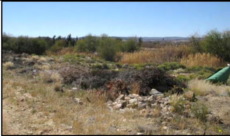
Figure 21: The section of the pipeline next to the water course from the N14.
