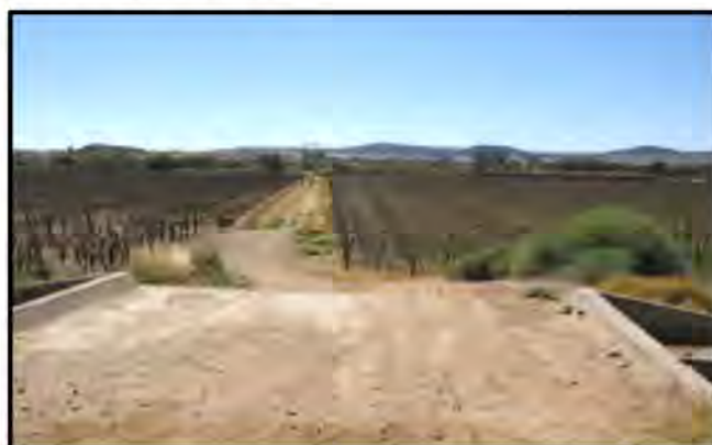
Figure 14: The proposed pipeline route will follow existing roads. This is the last section of agricultural land towards the banks of the Orange River, looking from south to north and towards the Orange River in the background.
