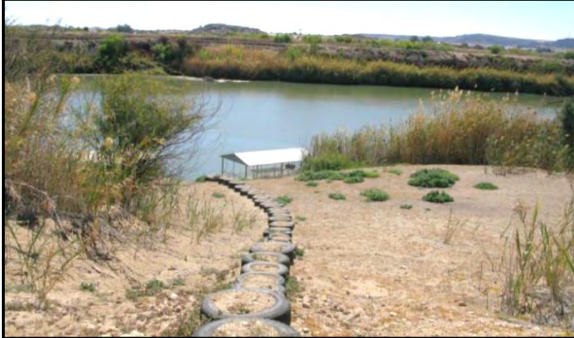
Figure 17: The proposed pump station location looking from the south towards the Orange River. Note the disturbance footprint.
