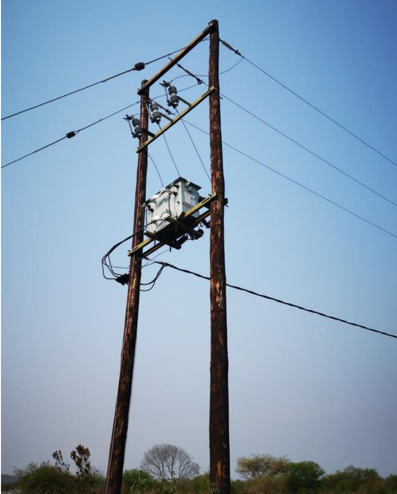
Figure 12 Electrical powerline in vicinity
