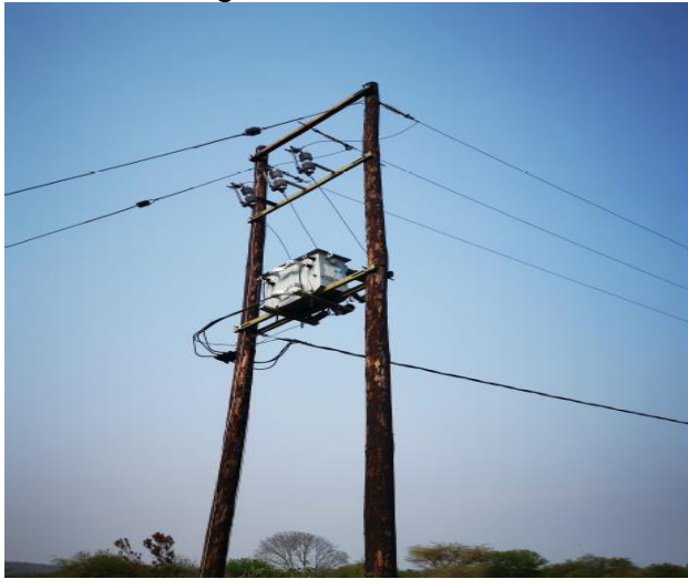
Figure 2 Existing Transformer and MV feeder line
