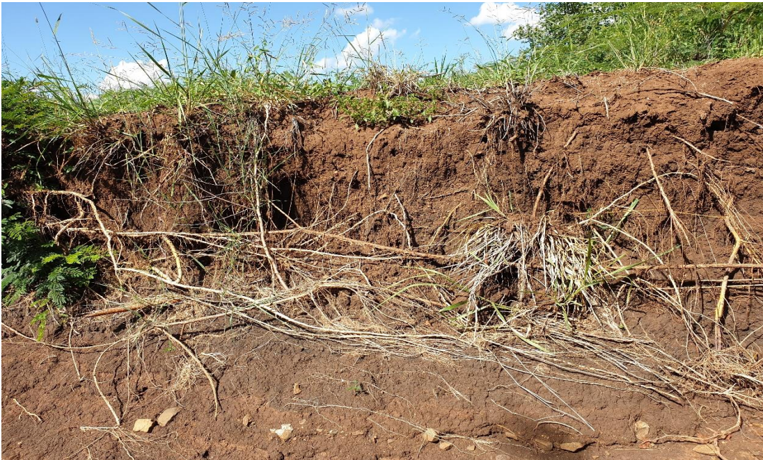
Photo 4: shows in side of the existing non perennial stream.
