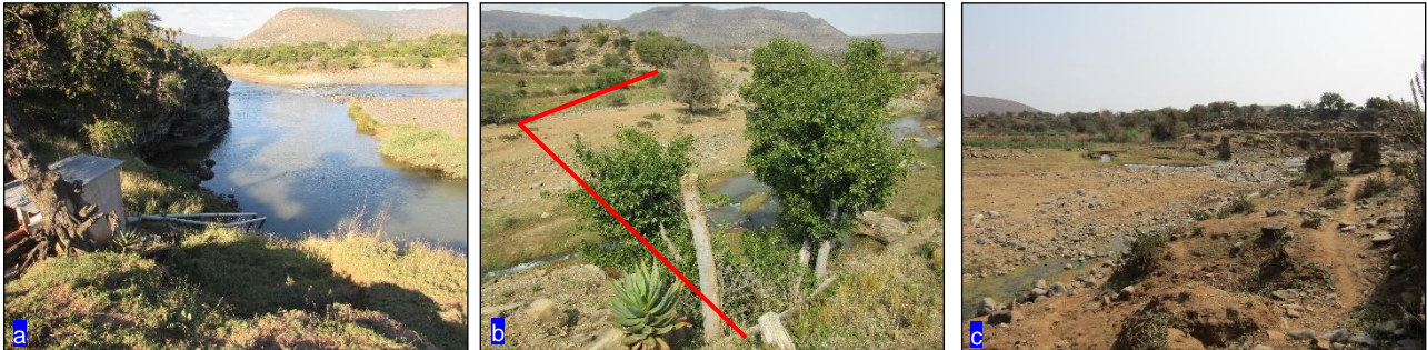
Figure 6: (a): Photograph showing the old dilapidated abstraction point. (b): View looking along the length of the Block 1 siphon from the inlet. (c): View of the river at the Block 1 siphon site.
