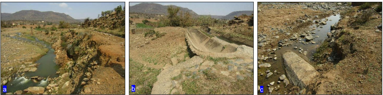
Figure 7: (a): View of the existing canal embankment near the Block 1 siphon site. (b): Evidence of erosion damage to the existing canals. (c): The existing siphon on the site to be replaced.
