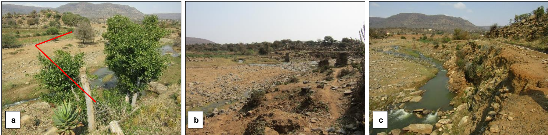
Figure 4: (a) View look along the length of the Block 1 siphon from the inlet; (b) View of the river at the Block 1 siphon site; (c) View of the existing canal embankment near the Block 1 siphon site.
