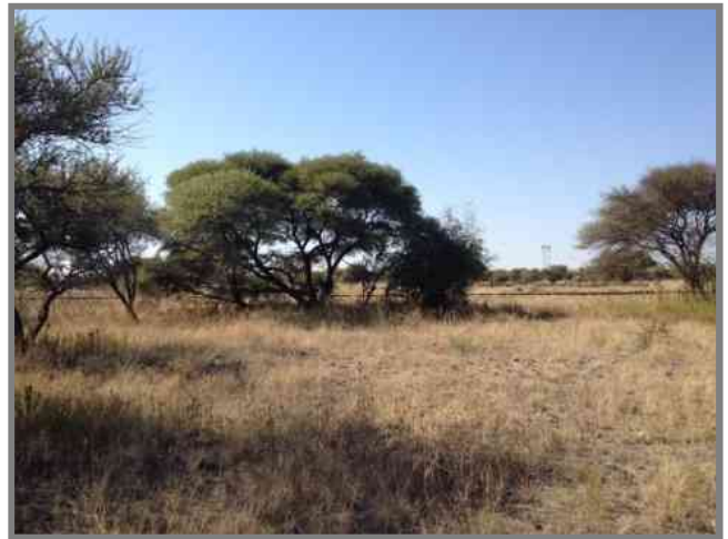
View east depicting Eskom transmission lines in the background
