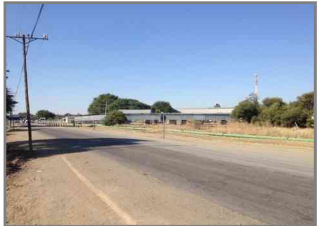
View east depicting mine workshops and administration structures
