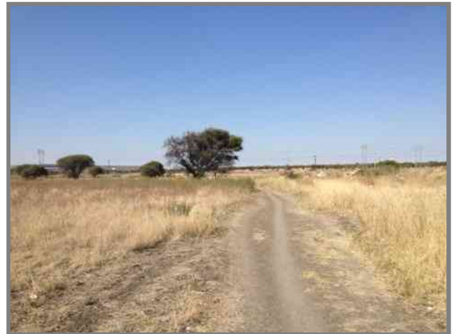
View east depicting Eskom transmission lines and mine access road
