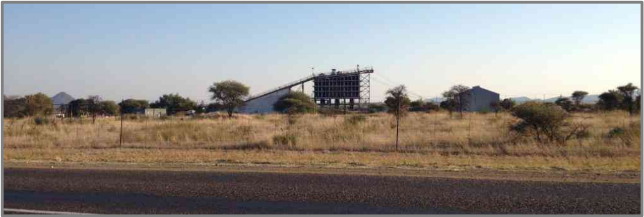
Figure 10: Derelect Mining Infrastructure
