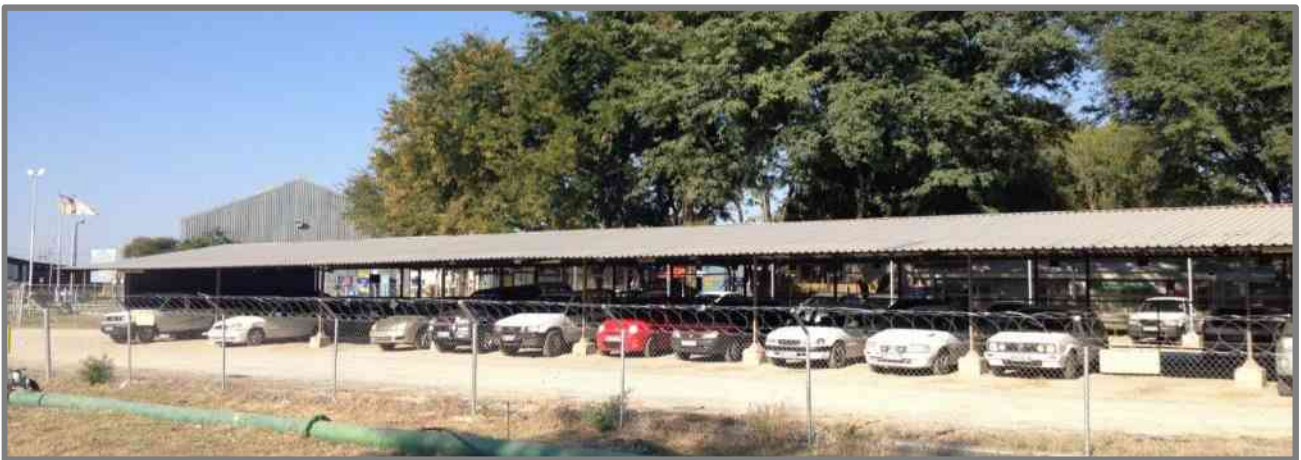
Figure 9: Existing Tumela Mine Workshops with effective incorporation of trees to create natural shade area
