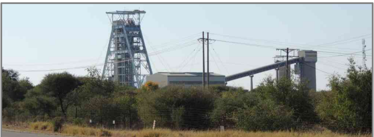
Figure 6: Existing Dishaba Amandelbult Mine shaft, Winching House and Silo infrastructure
