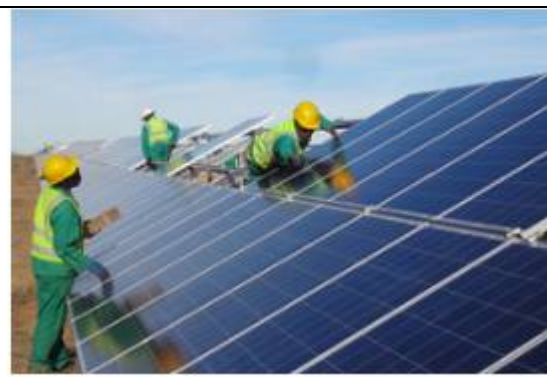
Figure 2.3: Picture of the installation of a typical PV array (75 MW plant in Kalkbutt South-Africa Source: PennEnergy)
