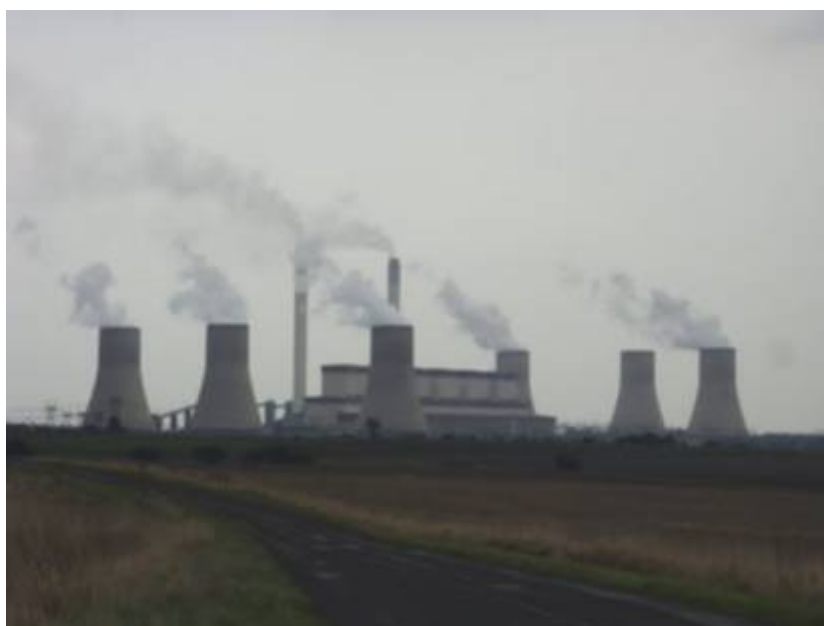
Figure 4.4: View of Tutuka Power Station. Note that the Tutuka PV Solar Energy Facility will be seen largely against this industrial backdrop
