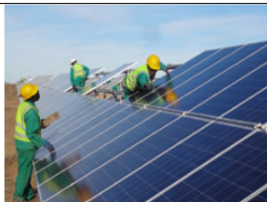
Figure 2.5: Picture of the installation of a typical PV array (75 MW plant in Kalkbutt South-Africa Source: PennEnergy)
