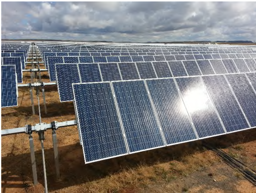
Figure 2.8: The support structures elevate the PV panels and allow for single axis tracking of the sun for increased efficiency (Source: SAPVIA)
