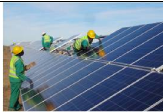
Figure 2.3: Picture of the installation of a typical PV array (75 MW plant in Kalkbutt South-Africa Source: PennEnergy)
