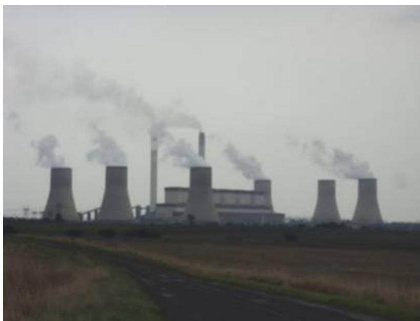
Figure 4.4: View of Tutuka Power Station. Note that the Tutuka PV Solar Energy Facility will be seen largely against this industrial backdrop
