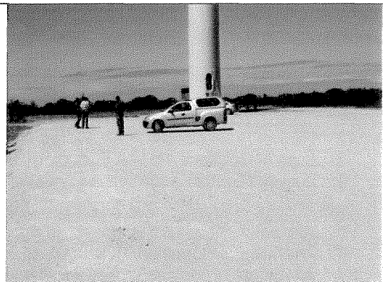
Figure 5-37: Example of typical wind turbine footprint (including lay down area and turbine footprint).
