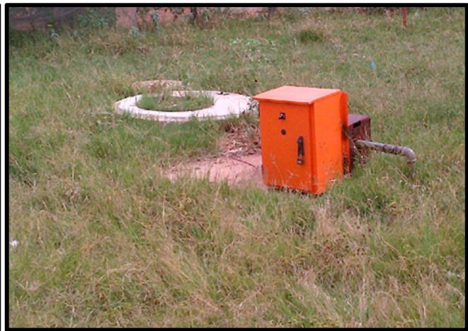
Figure 8: Borehole at Driefontein
