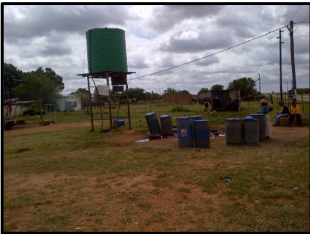
Figure 7: Elevated water Tank at Driefontein
