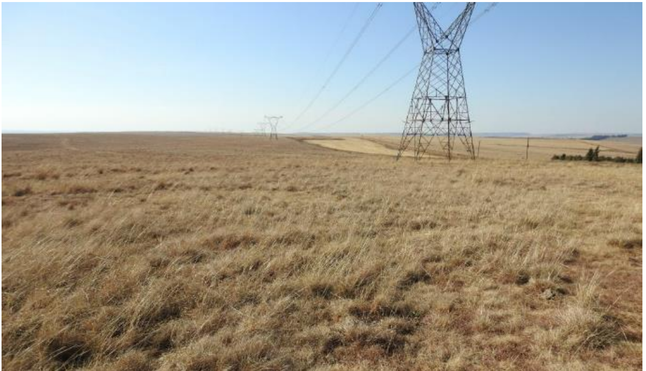
Figure 5: High voltage lines
