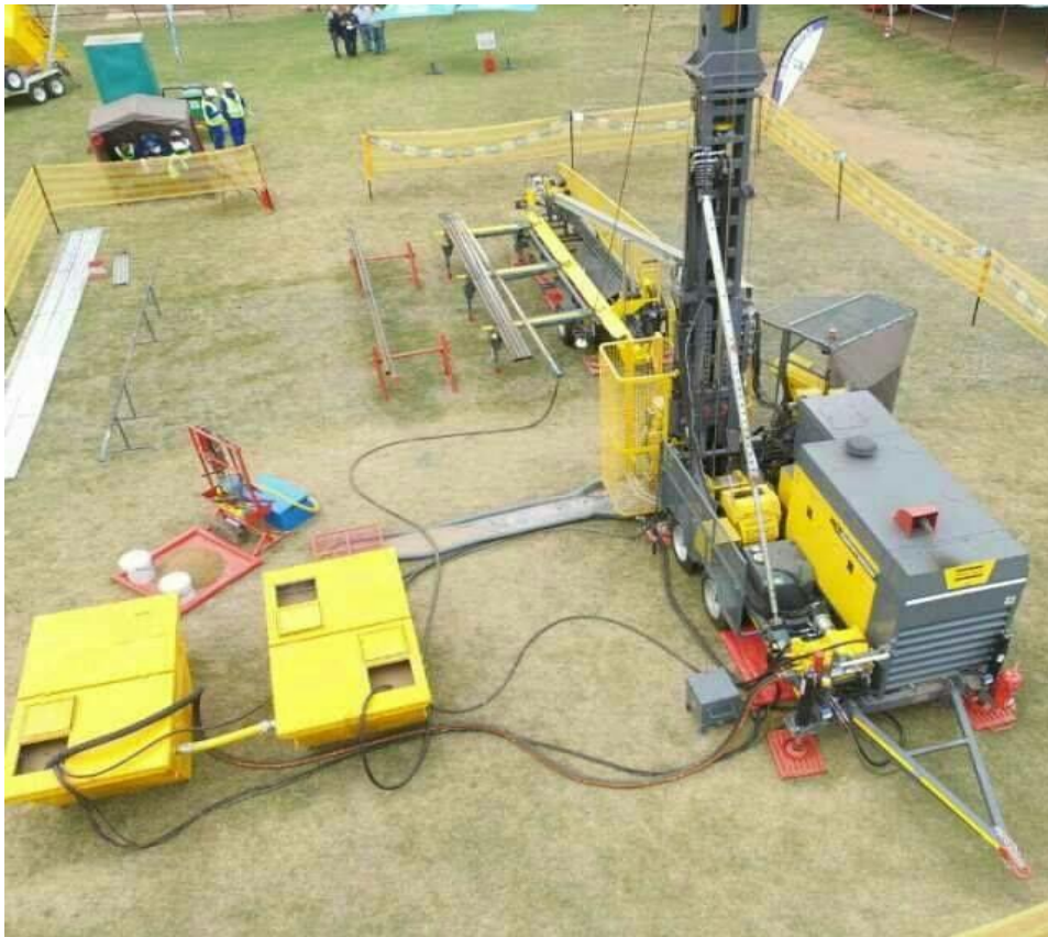
Figure 7: Typical examples of drill rig site
