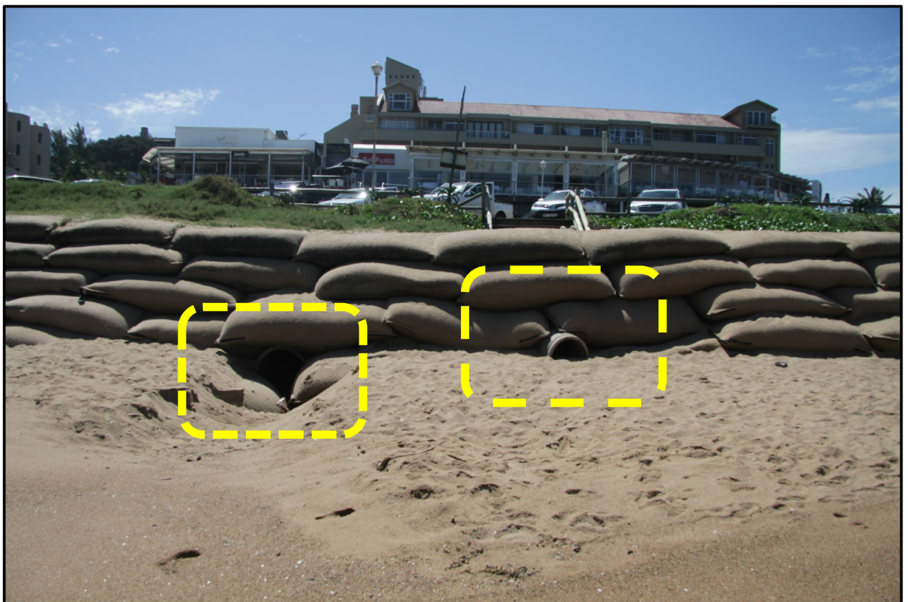
PLATE 7-3: The existing stormwater outlets which become blocked by beach sand and which will be abandoned.
