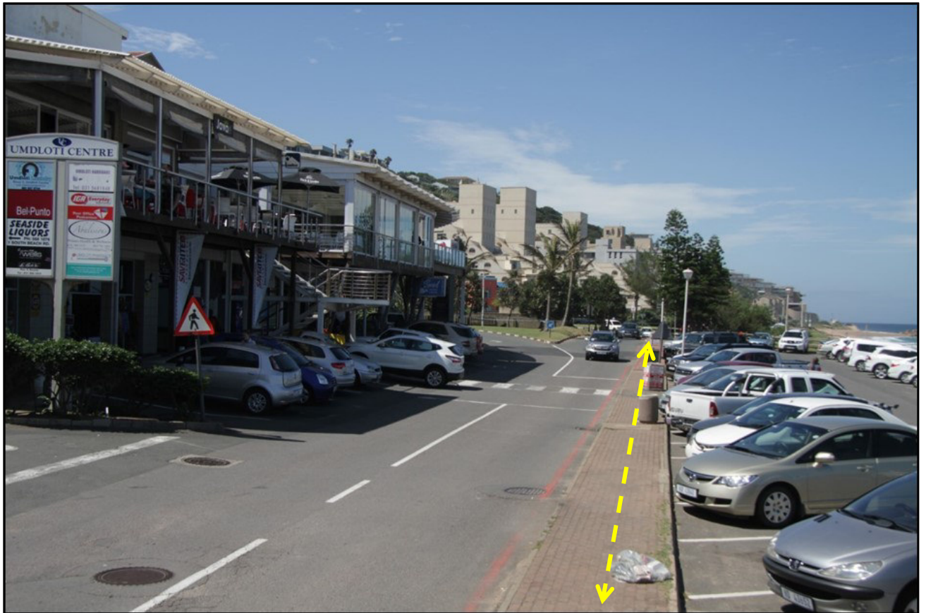
PLATE 7-2: The Umdloti Centre and parking lot adjacent to the proposed stormwater infrastructure.
