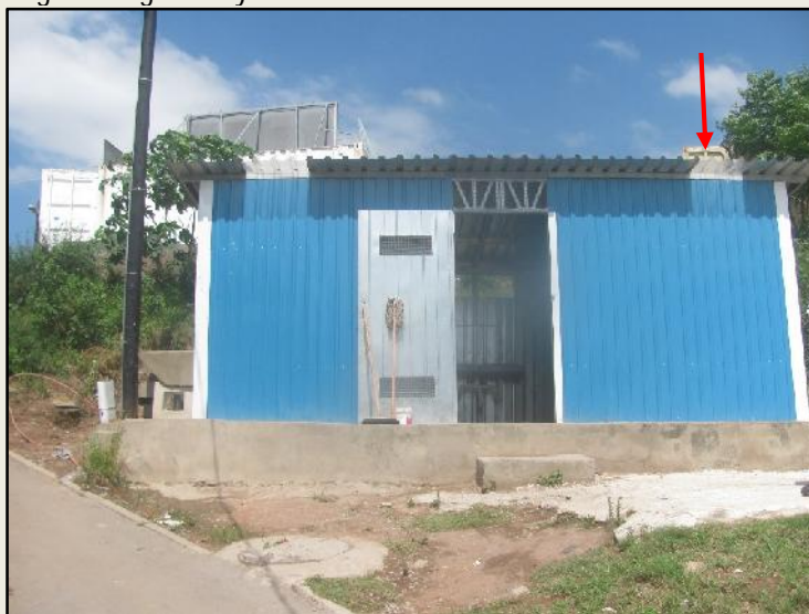
Figure three: CAB showing translucent sheets used on the roof
