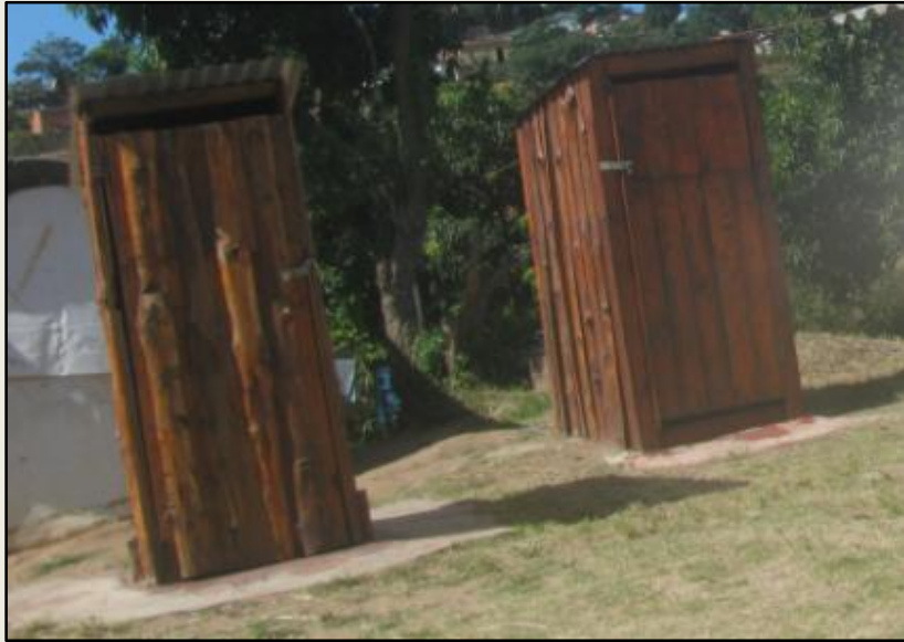
Figure three: VIP toilets are used when a connection to the sewerage system is not available
