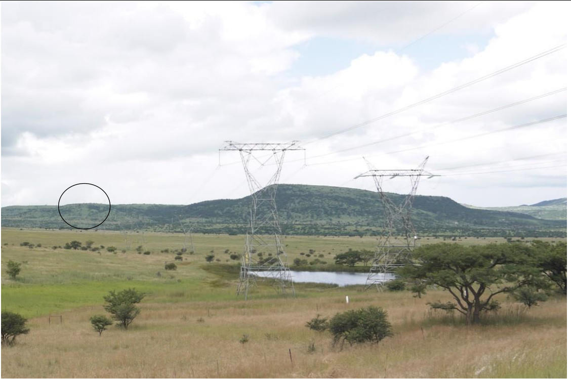
Plate 11 - Existing 400kV overhead transmission lines. Clearance of the servitude is the most obvious landscape change at a distance (approximately 5-7km)
