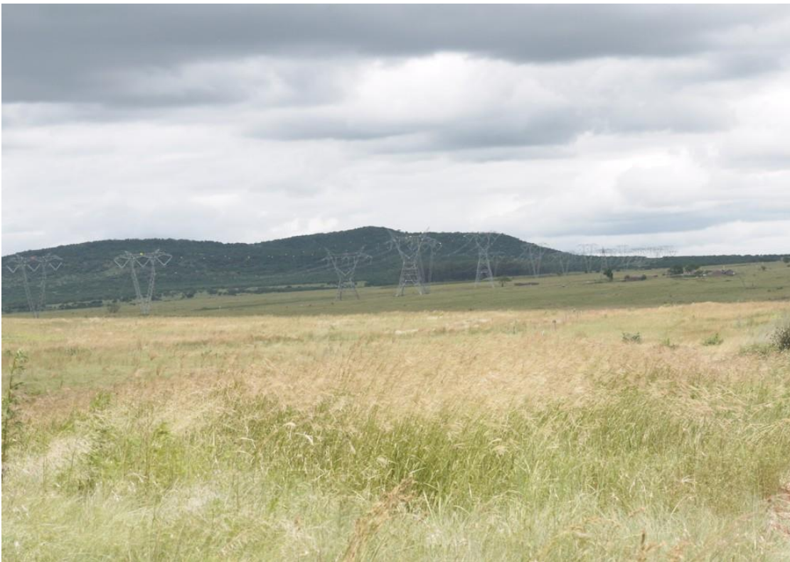
Plate 10 - Existing 400kV overhead transmission lines, obvious in the landscape at a distance of 1km to approximately 3-4km. Set against the dark landscape backdrop the towers are more obvious than when set against a lighter coloured sky
