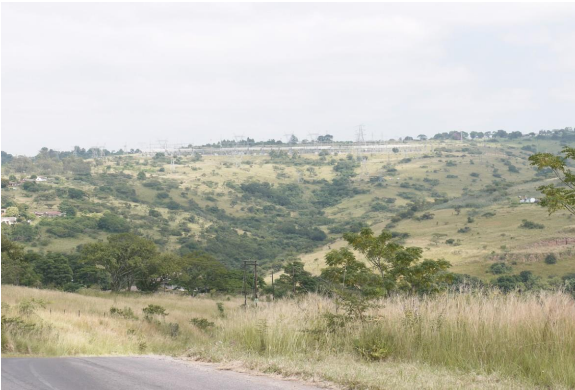
Plate 13, Distance view (1.5-2.0km) of the existing Hector 400kV Sub Station near Hammersdale.
